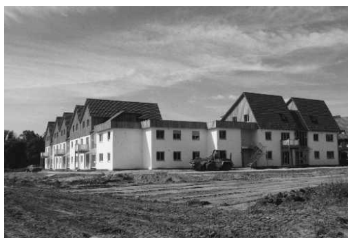
Figure 1 - View of Buildings
